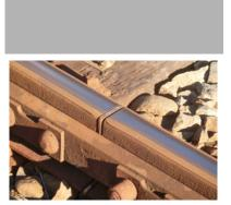
Explain how the addition of a small gap between sections prevents the bending of the track on hot days.
